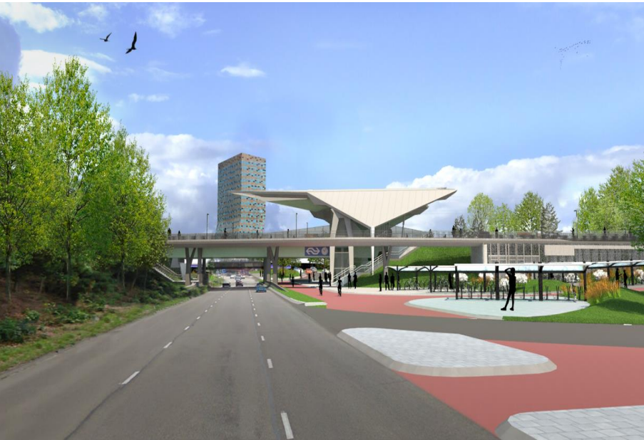
Station Goffert, the Netherlands
